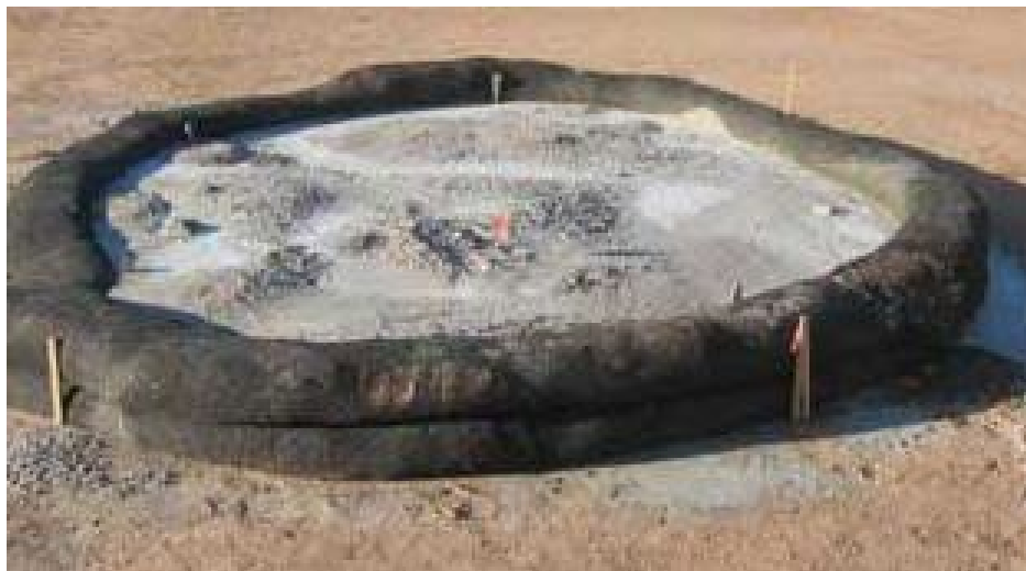
FIGURE 3.18 Typical Compost Sock Washout Installation
