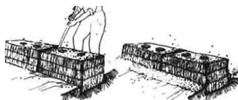
3. WEDGE LOOSE STRAW BETWEEN BALES
