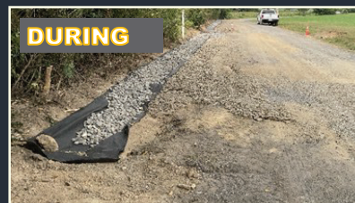
Installing buried drainage pipe to carry runoff water away from roadway
