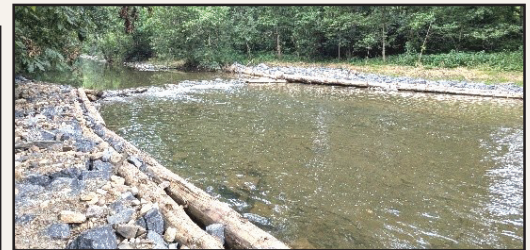
LEFT: The nearly completed log-framed cross vane with rock throat directs flow to the center of the channel.
