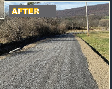
Completed DGR project on Robertson Road
