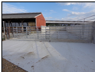
Recently completed stack pad
