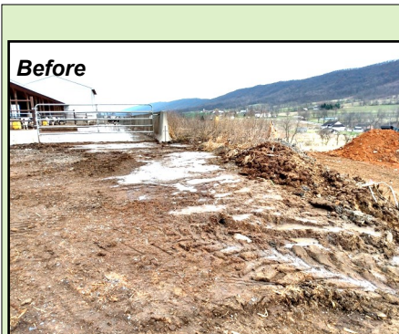
Above: Runoff from the barnyard. Manure was leaking through the jersey walls and had formed a small pond that would overflow and run through the field.
