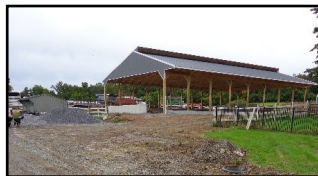
Recently completed animal heavy use area and stack pad
