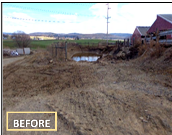
BEFORE AND AFTER Manure storage and transfer system completed using ACAP funding
