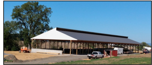
Roofed compost bedded pack and manure stack pad under construction
