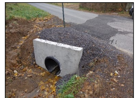
The newly installed 24-inch culvert
