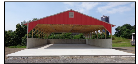
A completed roofed manure stack pad.
