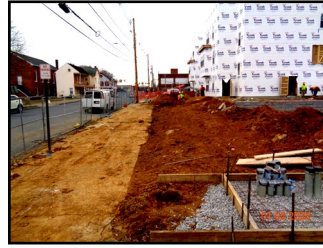
ABOVE: E&S controls in place during construction
