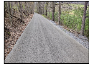
Brethren Church Road, Lurgan Township - With Driving Surface Aggregate being installed
