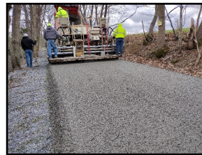
Brethren Church Road, Lurgan Township - With Driving Surface Aggregate being installed
