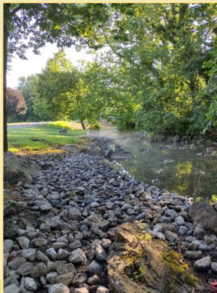
After a few structures had been placed, noticeable changes in the stream depth and flow were already observable, meaning that the structures were doing their job.
