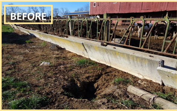
BEFORE photo shows manure leaking from a barnyard and entering a culvert pipe
