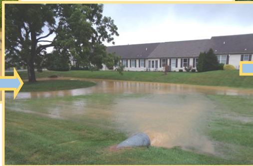
Example of what can happen when E&S controls are not properly installed or maintained. This sediment-laden water eventually affected the Conococheague Creek.
