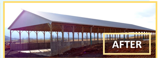
AFTER: To address the resource concerns, a liquid manure tank was designed and installed as well as a stack pad for bedding and solid material not suitable for the tank.
