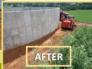
AFTER: To address the resource concerns, a liquid manure tank was designed and installed as well as a stack pad for bedding and solid material not suitable for the tank.
