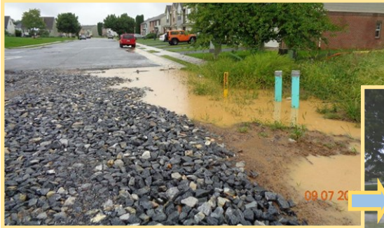
Example of what can happen when E&S controls are not properly installed or maintained. This sediment-laden water eventually affected the Conococheague Creek.
