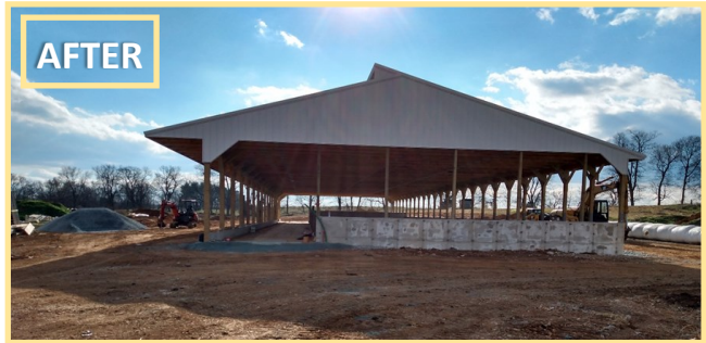
AFTER photo shows a bedded pack and stack pad nearing the end of construction. Both were designed to address the manure and barnyard concerns.
