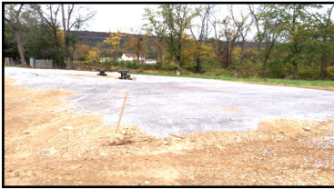
Animal heavy use area in early stages of construction. Note the nearby vegetated filter strip in place to reduce pollutant loading to the creek
