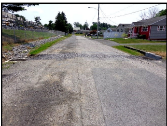
Pipe replacement on Harrison Drive
