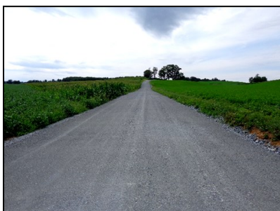
Quincy Township, Green Corner Road: Driving Surface Aggregate placed
