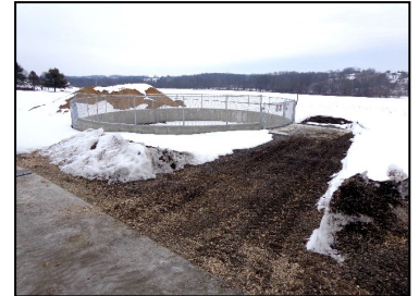
Completed reception pit and circular manure tank 2020
