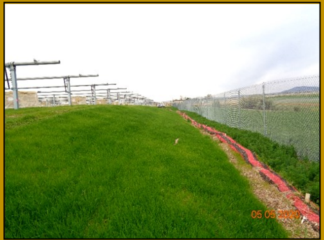
This photo accurately demonstrates the effectiveness of erosion control matting and why the District emphasizes its use. This slope was stabilized with erosion control matting unlike the photo to the left. You can see how effective the matting is at establishing vegetation and holding disturbed soils in place.
